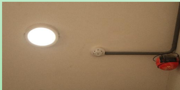
Example of Energy Efficient Appliances Usage: Use of LED lighting and lamps with light detection (Shaheed Benazir Bhutto University, Shaheed Benazirabad)
